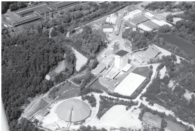
Fig. 3: The Rhineland-Palatinate Company EKW GmbH, Germany, with its own raw material deposit luting sand (“Eisenberger Klebsand”) and high-end production facilities
